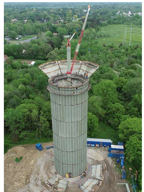
Site construction of Genesee County's newest elevated water storage tank.
