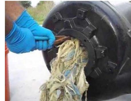
**“Flushable” wipes do not break down. The resulting mess- like pictured above- clogs plumbing systems and blocks sewer lines.**
